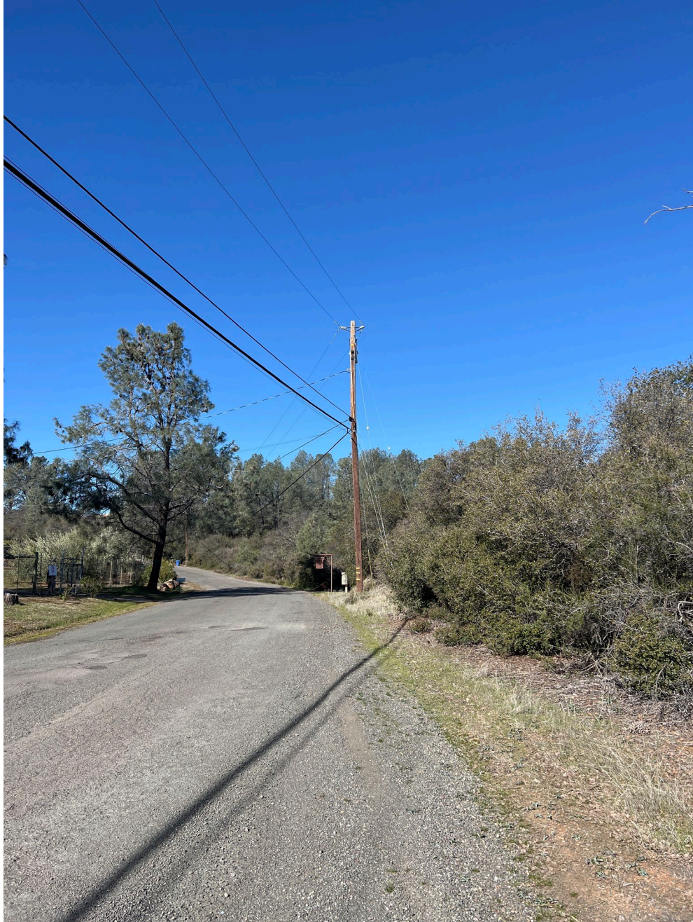
Point A: Conditions prior to mastication, note the narrow width of road corridor.
