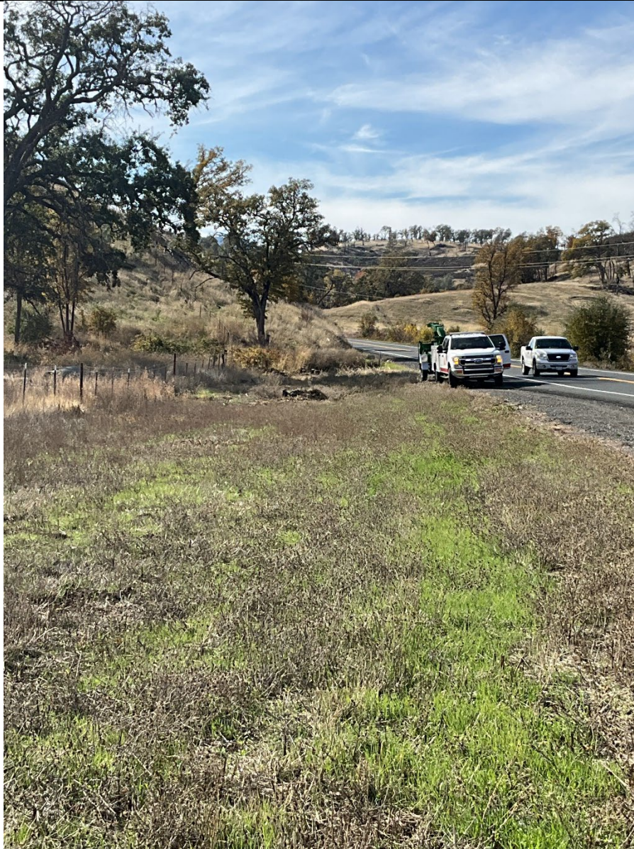
After: Typical roadside conditions north of Middletown post-treatment.
