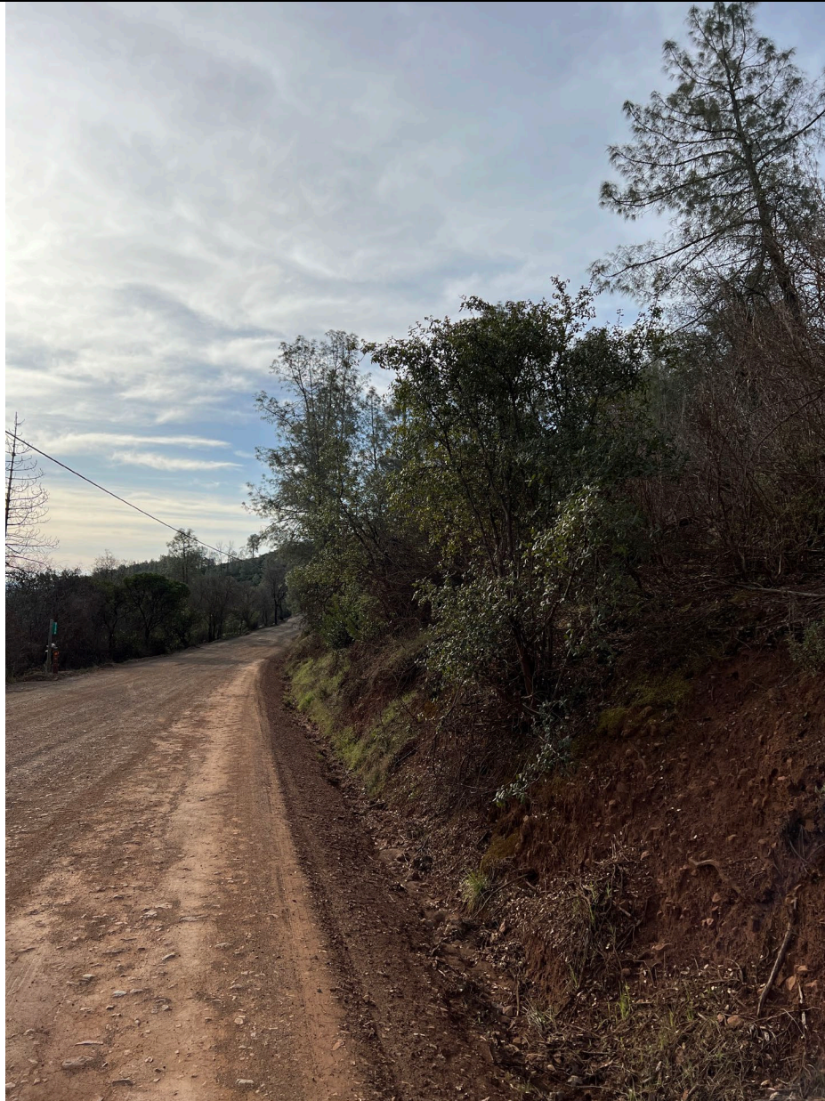
Point B: Typical conditions before mastication, note vegetation encroachment to the roadside.
